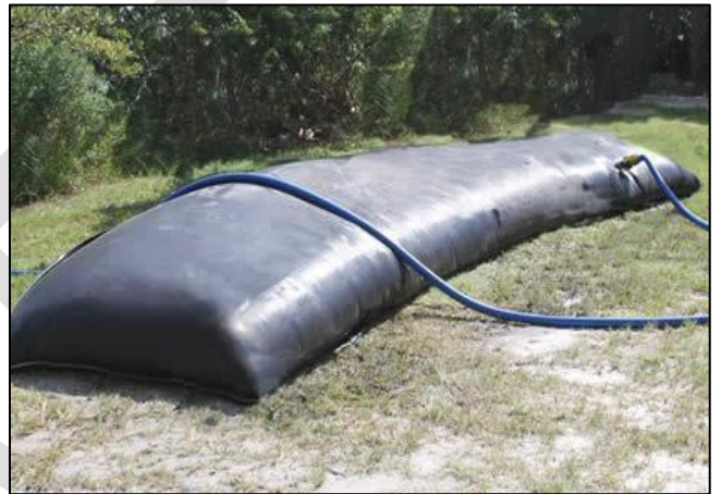
Photo 8. Sediment dewatering bag.
