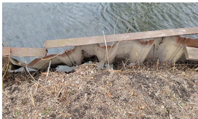
Photo 6. Seawalls no longer offer shoreline protection.
