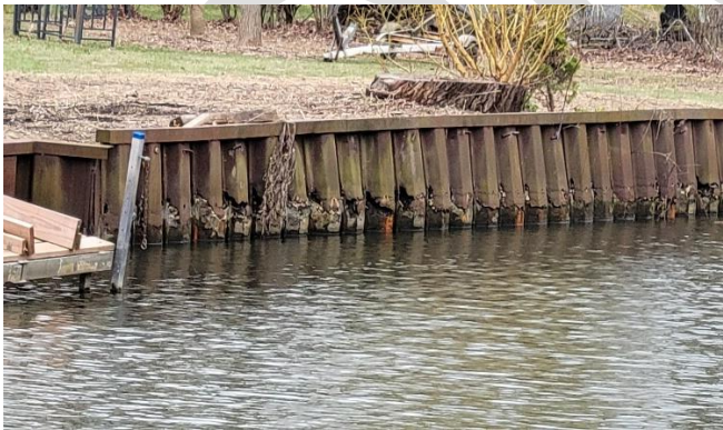
Photo 3. Example of failing seawall on the channel.
