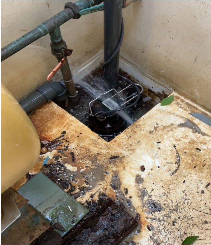
Photo 3 - Sump Pump in the Vault
